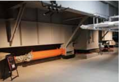
Seismic isolation equipment in Planet Saitama
